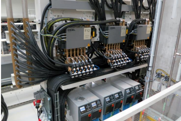
Compact integration: the production cells are equipped with e-flooms and temperature control units located on the sides and to the rear of the machine.
