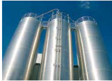
Outdoor raw materials storage silos
